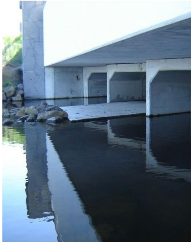
The box culverts were set in under the road verge, to reduce the length of the passage.
