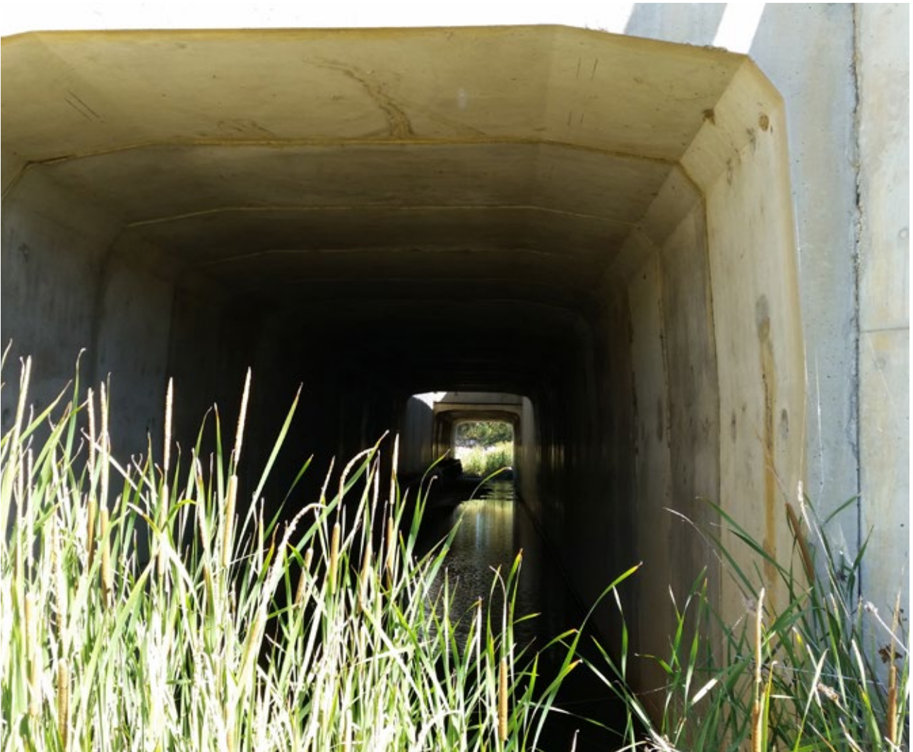
A large vent in the median strip improves conditions for Growling Grass Frogs in a long culvert under the Calder Freeway. Photos by Kathy Preece
