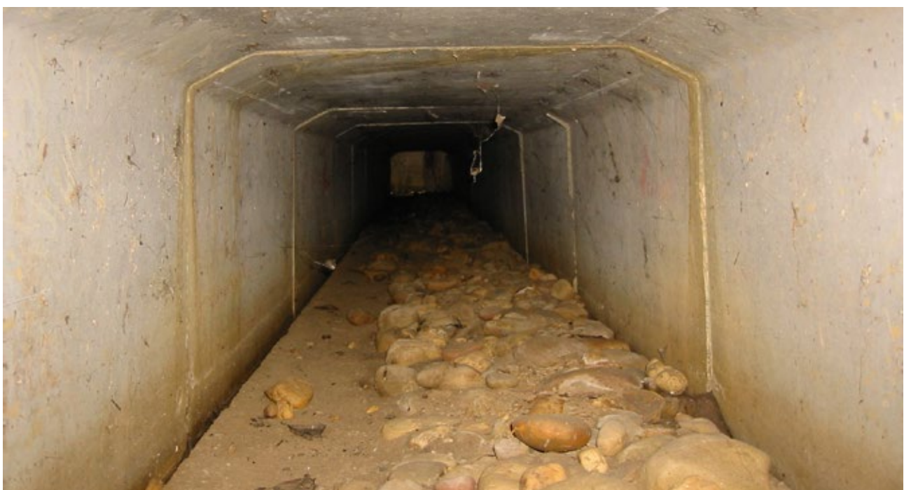
The conditions inside regular small box culverts are colder, darker and drier than outside, and there is no conclusive evidence that Growling Grass Frogs use them to pass under roads. Photo by Peter Robertson, Wildlife Profiles Pty Ltd
