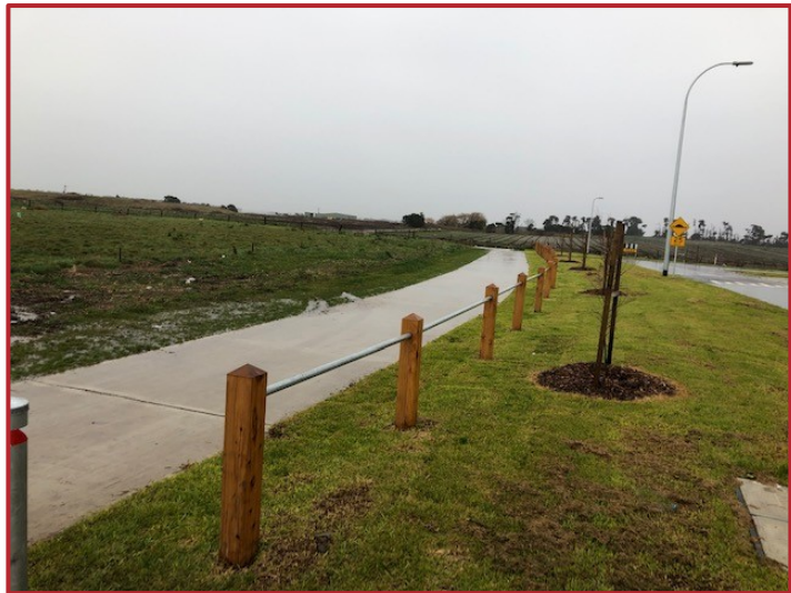
Figure 2: A post and steel rail fence constructed at a GGF conservation area (Credit: DEECA).
