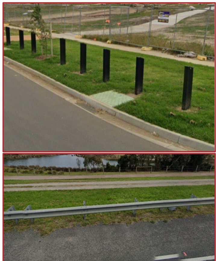
Figure 5: Examples of road reserve installations that may influence the need for boundary fencing if they are near the conservation area. A bollard streetscaping treatment (top), and a road barrier (bottom). (Source: Image capture © 2021 Google).
