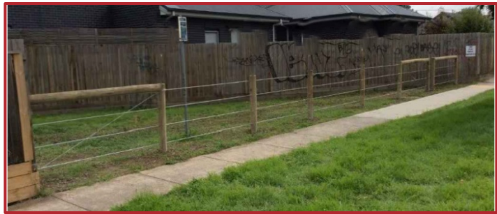
Figure 1: Example of the post and cable (four strand) fence style (Credit: Melbourne Water).
